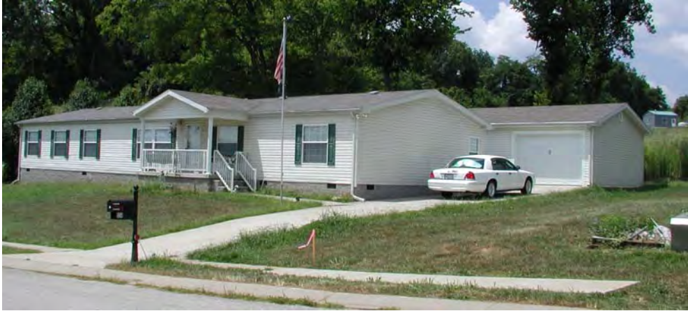
Figure 5.3: Manufactured Home With Post-production Porch and Attached Garage
