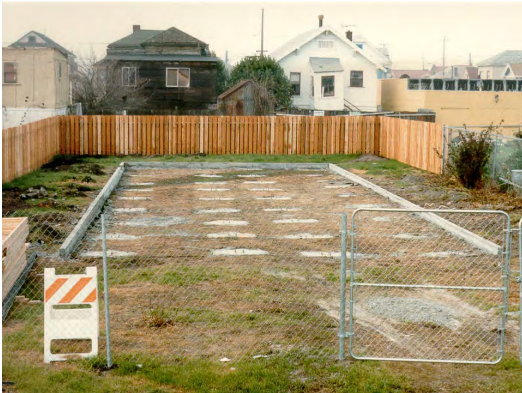
Figure 2.7: Foundation for a Manufactured Home Duplex
