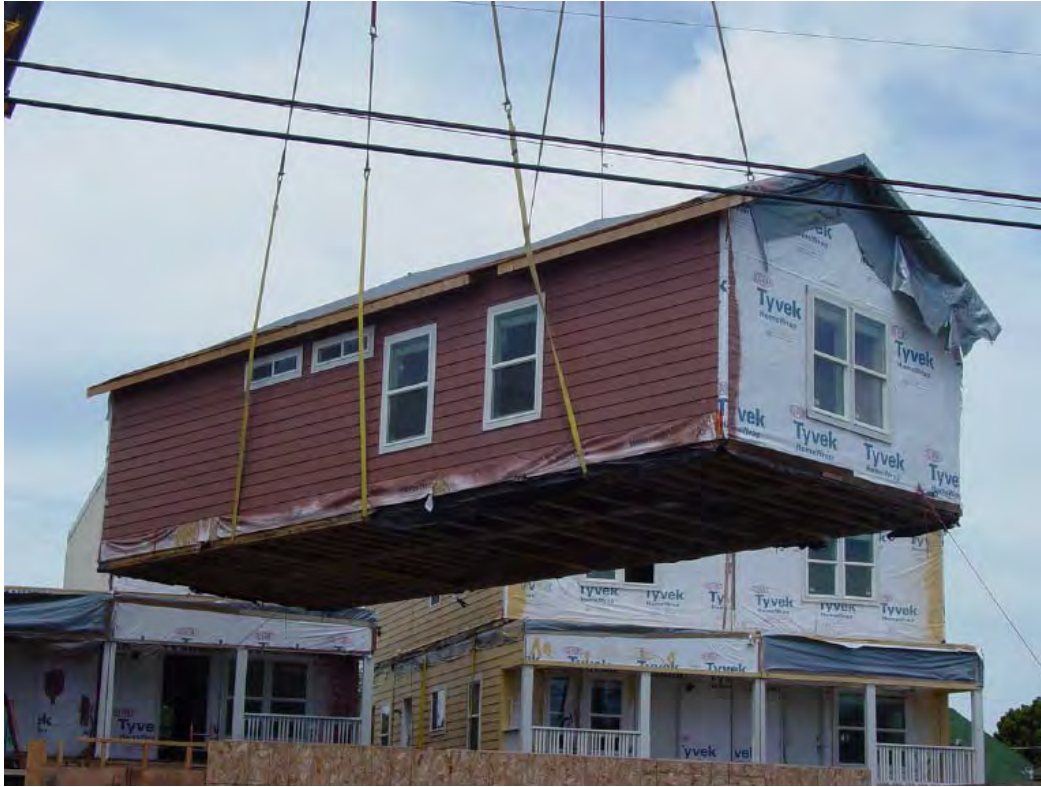
Figure 2.15: Crane Installation of HUD-Code Home
