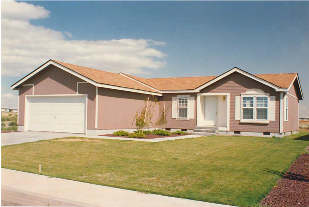
Figure 3.10: Manufactured Home on Infill Site in Pasco, Washington
