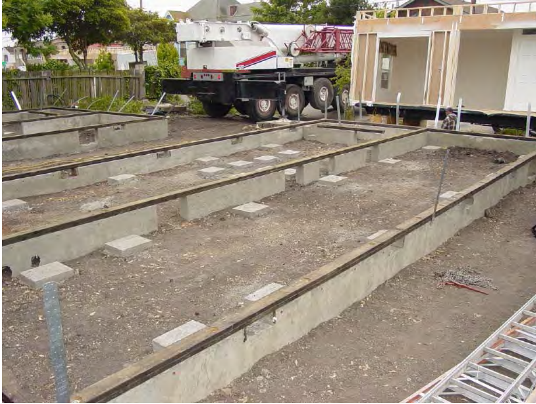
Figure 2.6: Foundation for a Two-story Manufactured Home
