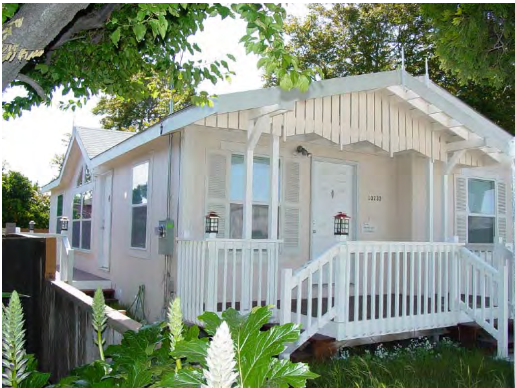
Figure 2.10: Carpenter Built Front Porch and Detailing on Manufactured Home
