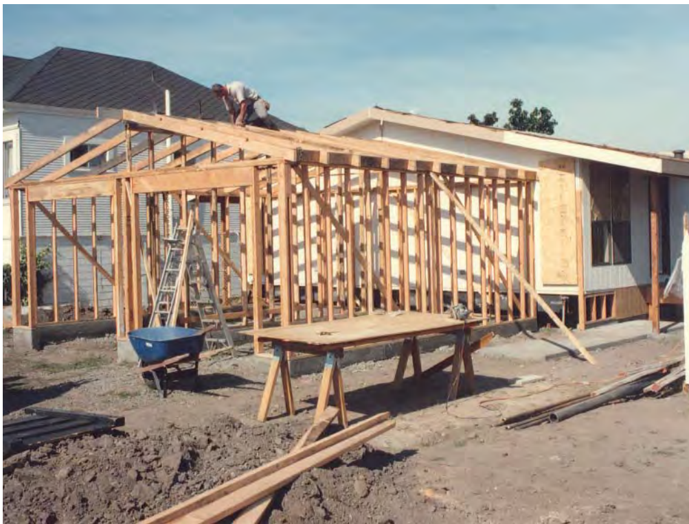
Figure 2.8: Garage Abutting Front of Manufactured Home
