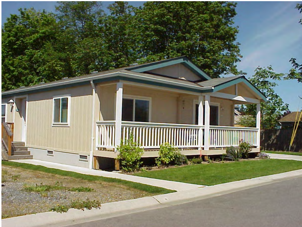
Figure 3.7: Manufactured Home in Thomas Place, Everett, Washington
