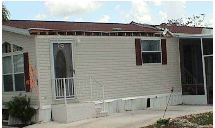
Figure 27. (Above) Typical damage to the eave of a home when a carport roof is blown away during a hurricane. About six square feet of area at the top of the wall was opened allowing entry of wind-driven rain.
