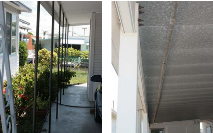
Figure 16. Left image shows typical old support system where pipe posts connect to small thin angle. Right image shows carport with replacement beam and 3" x 3" posts; note severely rusted bolts.
