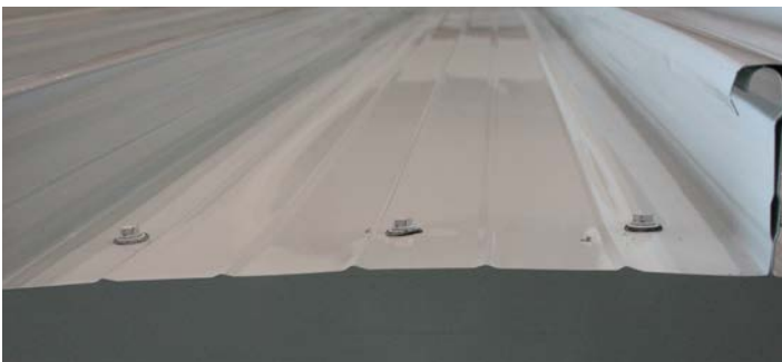
Figure 34. Initiation of panel connection failure at connections using small screws without metal/neoprene combination washers.
