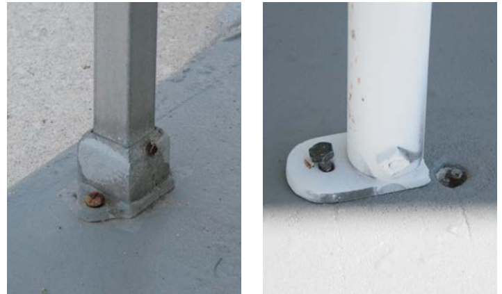
Figure 14. Other examples of poor post connections at base. Cast aluminum bracket (left) and broken bracket with dislodged screw (right). Note inadequate spacing of fasteners from each other.
