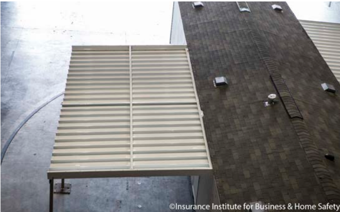
Figure 22. Single 2" x 4" beam across middle of pans to help resist uplift; 2" x 4" beam is supported at ends by 2" x 7" beams spanning ends of carport.
