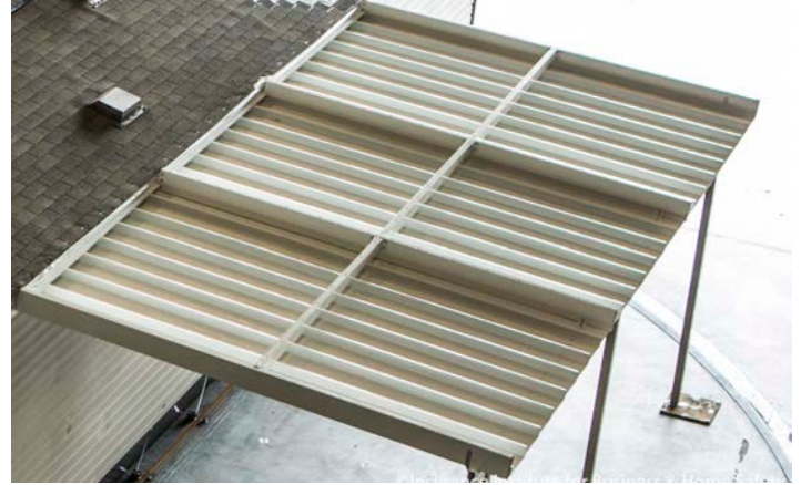
Figure 24. Modified retrofit with two additional 2" x 7" beams so each section of 2" x 4" brace only spanned 8'.
