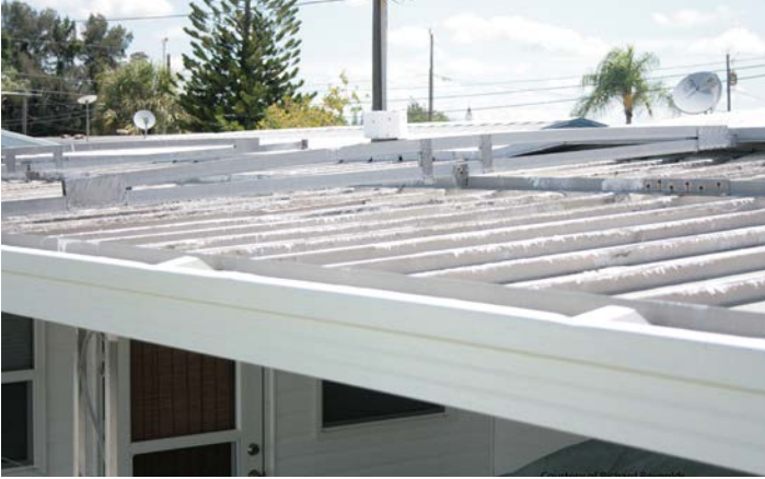
Figure 21b. Complex arch truss and brace system intended to prevent uplift buckling of roof pans.
